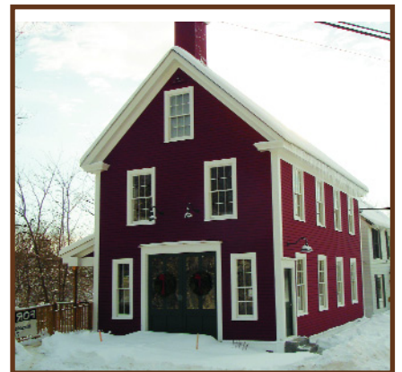
Historic firehouse Converted Into Office Spaces
